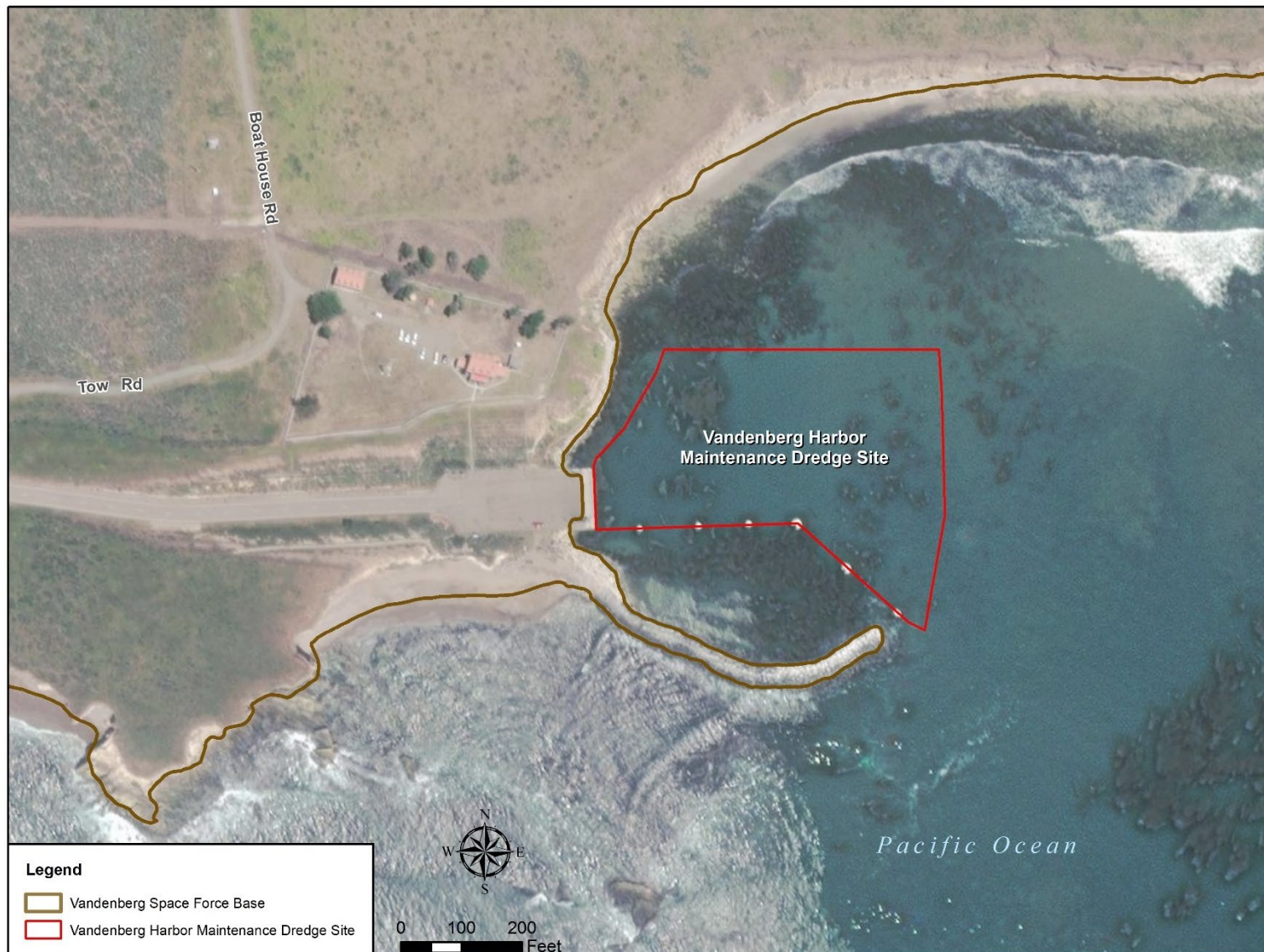
Figure 2-1. Maintenance Dredging Area
