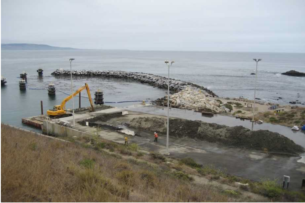
Figure 2-2. Dredging and Sediment Staging with 70-foot Crane
