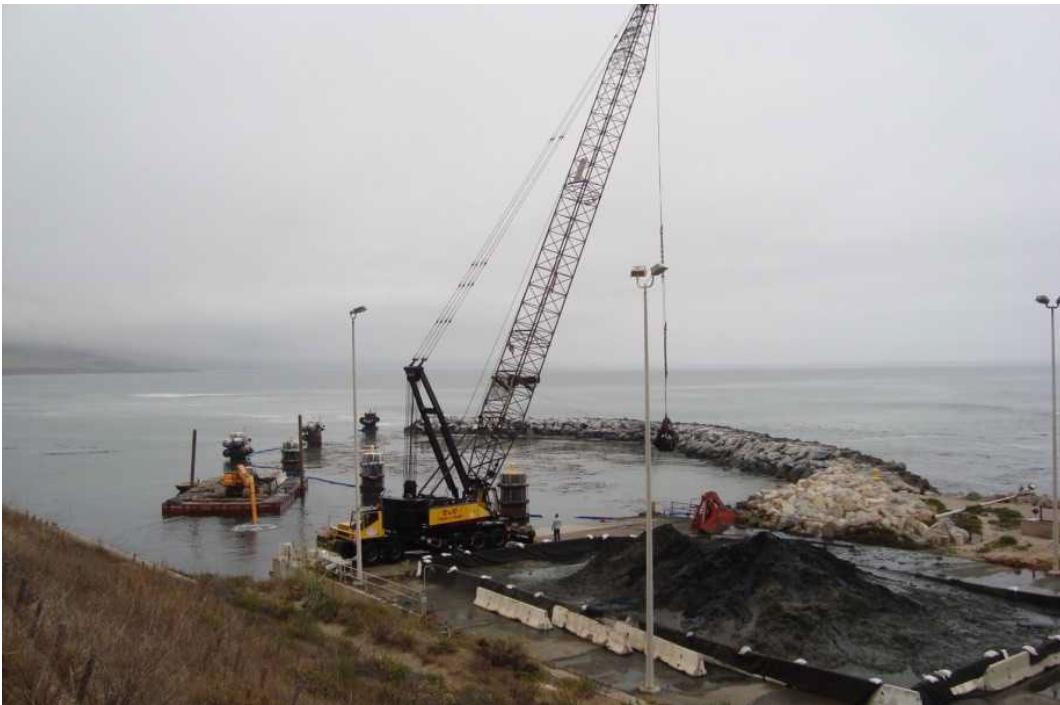
Figure 2-3. Dredging and Sediment Staging with 200-foot Crane
